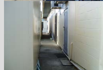
Existing cross-block links need improvement
